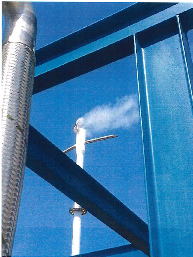
Hydrogen Vapor from Vent Stack
